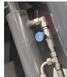
Figure 23. Throttling valve
